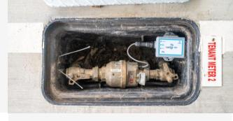
Multi Sensor Interface Chosen for its multi sensor interface that can connect to existing infrastructure and flow sensors at the same time
